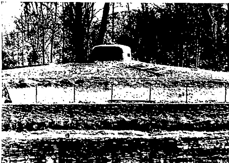
Figure 26.—Work with cupola, embanked.
