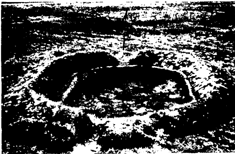
Figure 46.—Emplacement for antitank gun in flat terrain.
